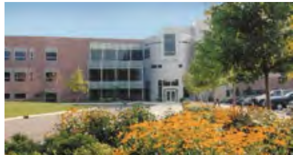
Parker Hannifin Corporation Headquarters Cleveland, Ohio
